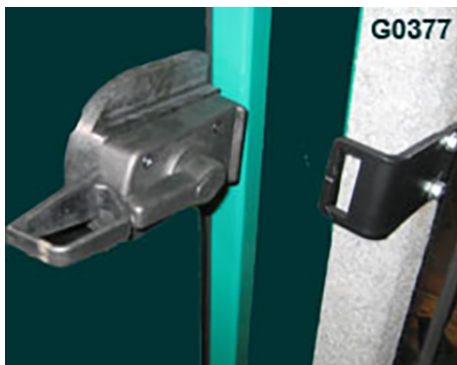
Fig. 91 Latch handle, emergency exit
