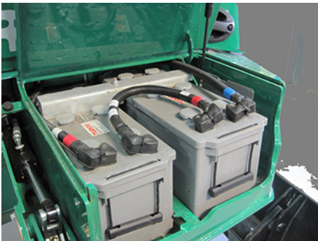
Fig. 142 Batteries in the right branch deflector
