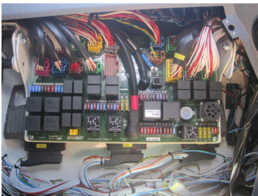
Fig. 146 Distribution box in cab
