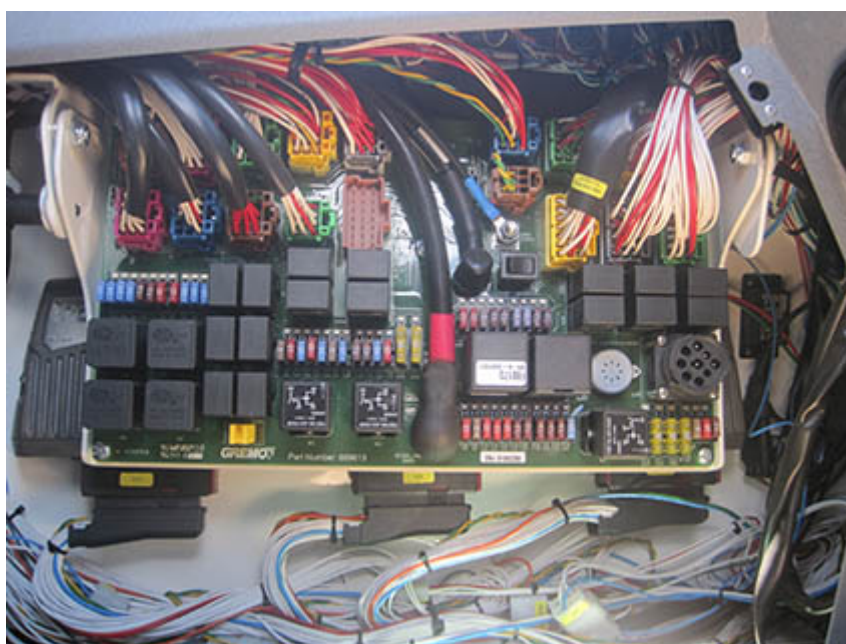
Fig. 138 Distribution box in cab
